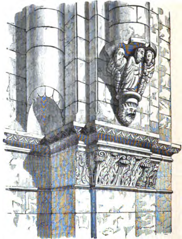
RESPOND, WESTERN ARCH OF CENTRAL TOWER, LOCHES.
